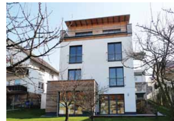
Covering four storeys, this two-dwelling building was designed by r-m-p architects, which has built a number of Passive House constructions in the local area of Schriesheim, Germany. Because of the sloped plot the basement is built out of concrete with external insulation. The other three storeys are constructed from timber and use internal insulation.
