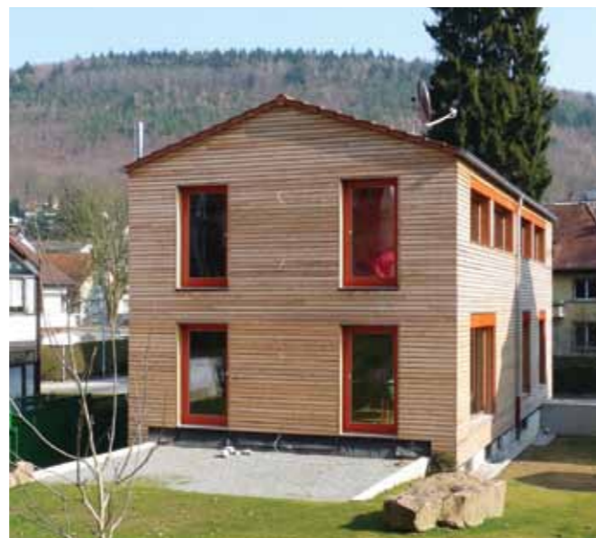
Located in Neckargemünd, Germany, this residential building consists of a ground floor concrete construction with a two storey timber living space encompassing the Passive House envelope. r-m-p architects designed the house to bridge the sloping ground between the front and rear elevations.
