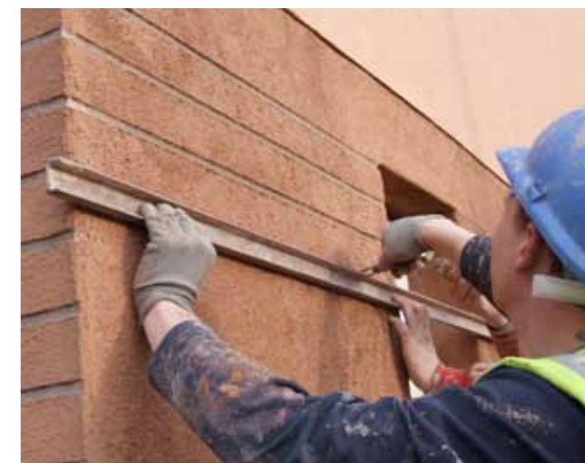
The External Wall Insulation being used in the trial
