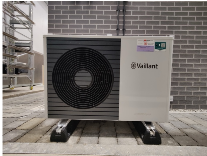
Figure 8. Vaillant ASHP External Unit
