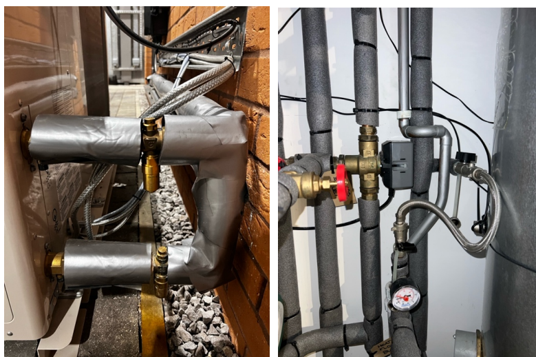
Figure 176. Left) Caleffi 108 series antifreeze valves. Right) Filling loop left in place
