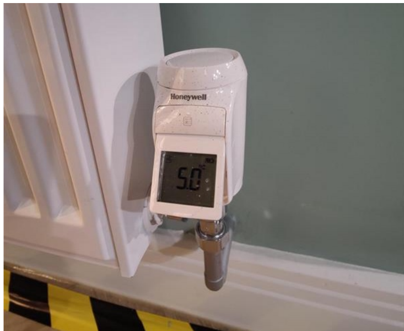
Figure 7. Honeywell TRV
