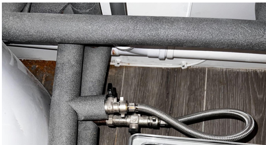
Figure 169. Filling loop should be removed post installation to avoid any possible cross-contamination
