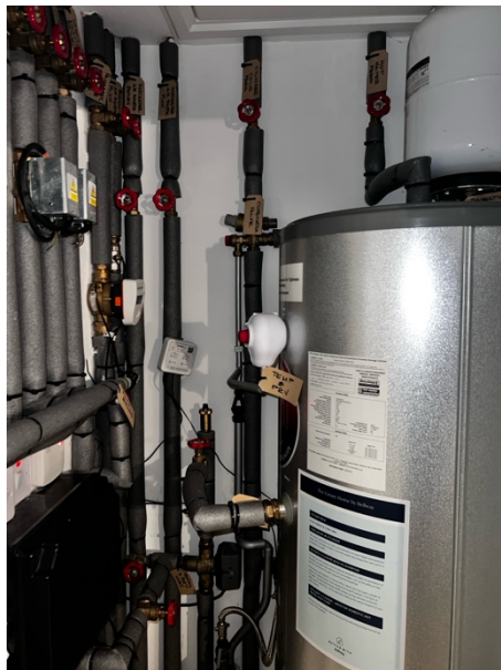
Figure 172. Cylinder without TMV protection
