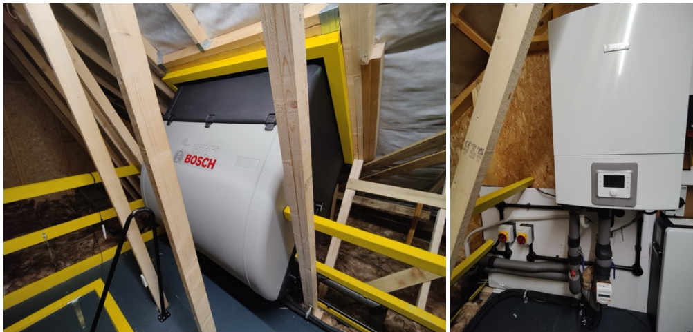
Figure 3. Worcester Bosch ASHP Hydrotop (Left), Internal Unit (Right)
