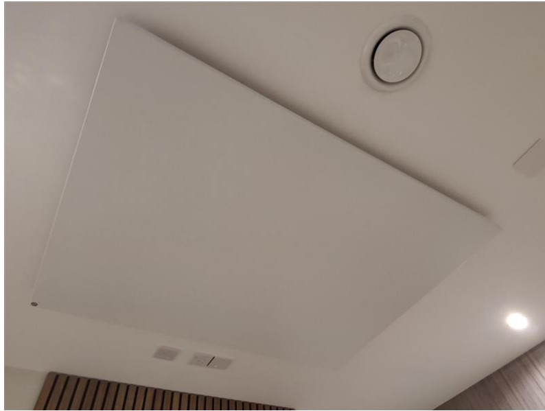
Figure 5. Wondrwall infrared panel
