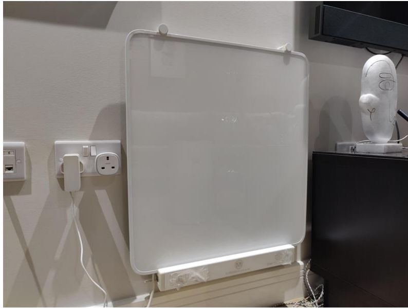
Figure 6. Ambion infrared panels
