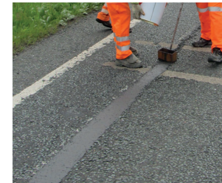
SAFETRACK® INLAID ROAD REPAIR APPLICATION
