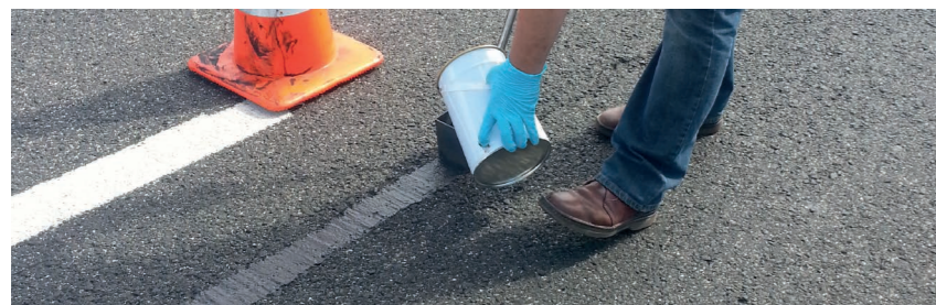
SAFETRACK® CRACK INFILL APPLICATION
