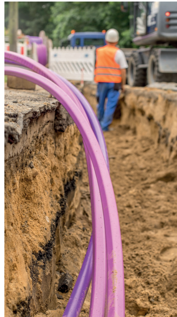
HIGHWAY REINSTATEMENT WORKS
