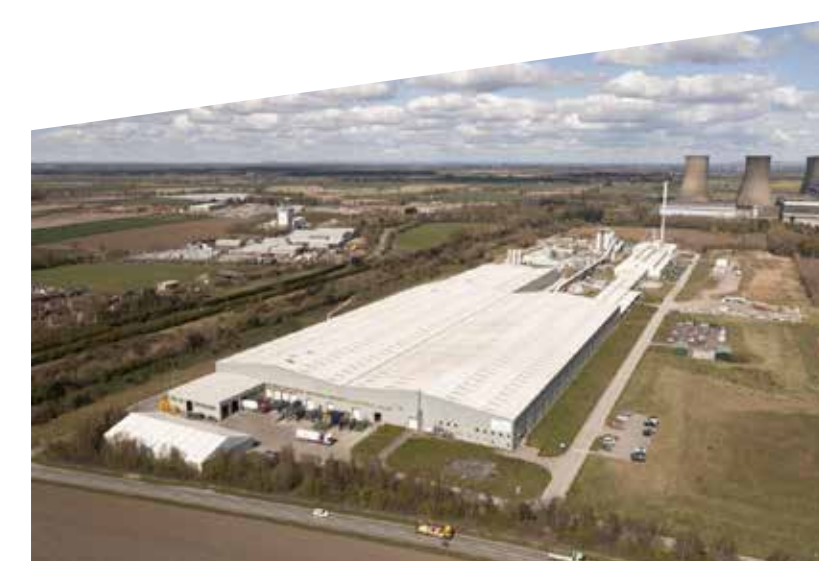
FLOAT GLASS PRODUCTION, YORKSHIRE
