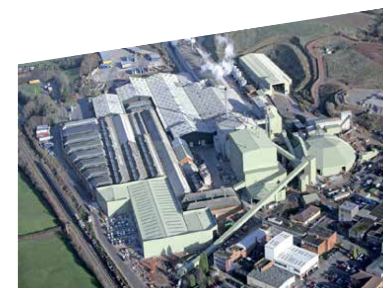
EAST LEAKE, PLASTERBOARD
